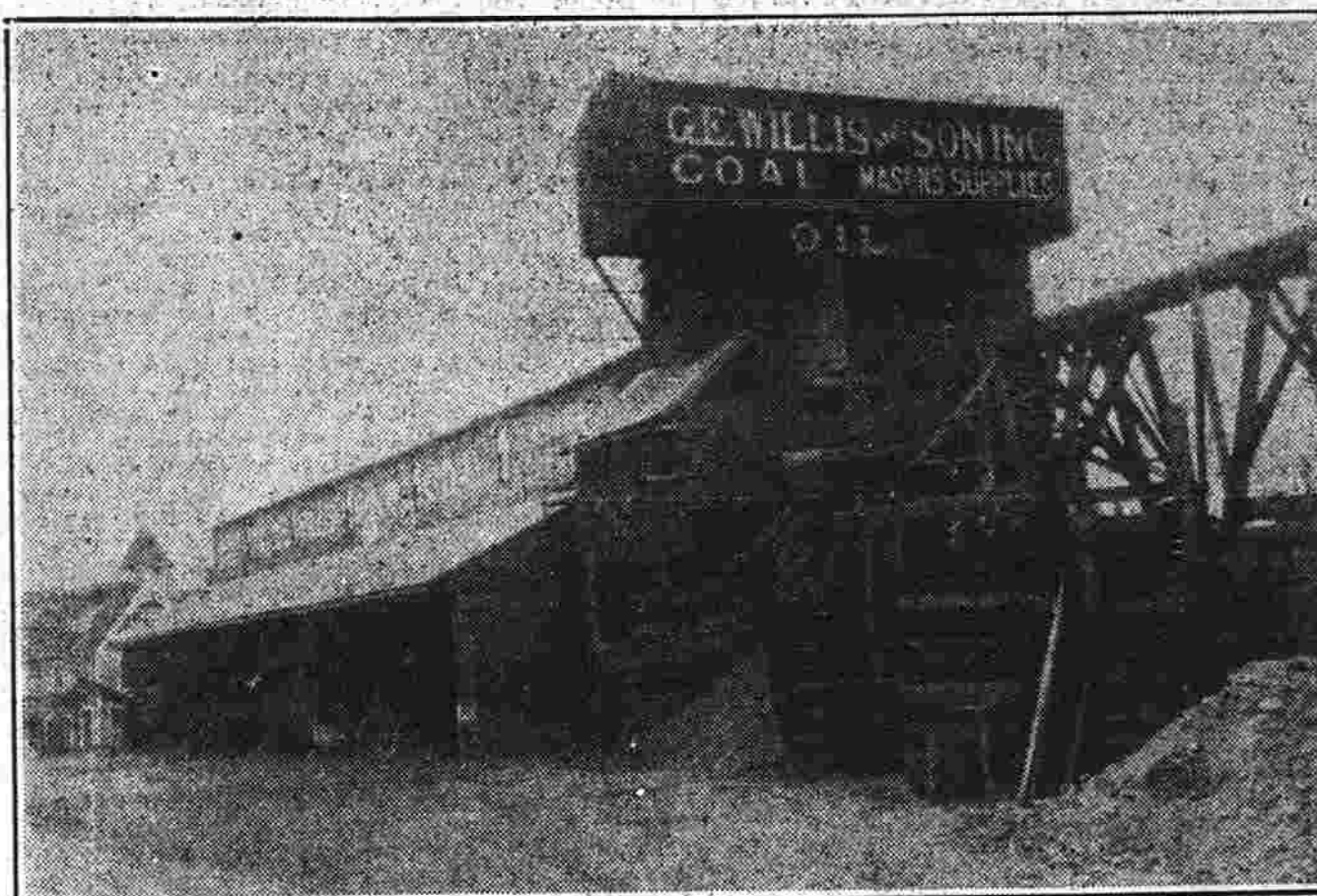
Our coal storage yard is not to be excelled anywhere for capacity or equipment. Coal in cars is brought to the base of the tower, brought up by bucket elevator to the hopper at the top and distributed by conveyors throughout the length of the shed. We have handled Old Company Lehigh for many years because we know its quality. All coal loaded in trucks by screened conveyors.
